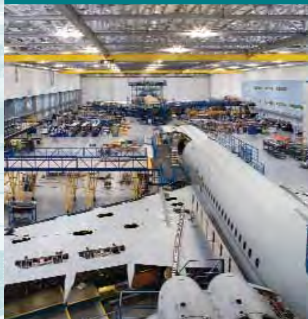
St Athan's super hangar before closure
